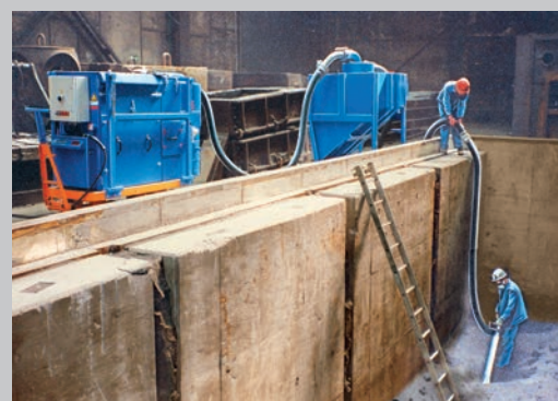
Vacuum extraction of blasting material in a dry dock
