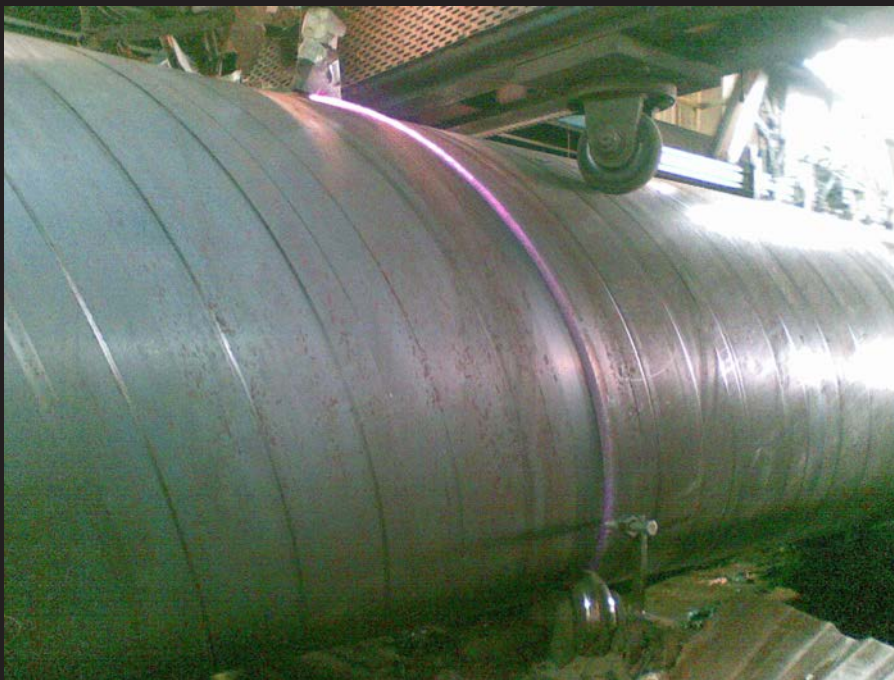
Extraction of welding powder during spiral pipe welding
